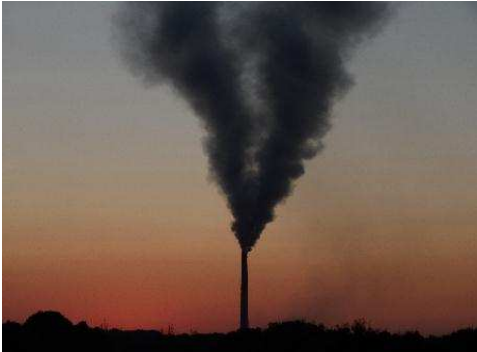
1.8 GW Ladyzyn thermal power plant at dusk. Photo: NECU archive
