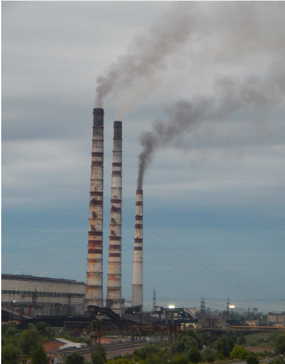
50 year-old 2.3 GW Burshtyn thermal power plant. Photo: Oleg Savitsky
