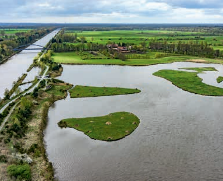
Shallow water zone at Mannhausen
